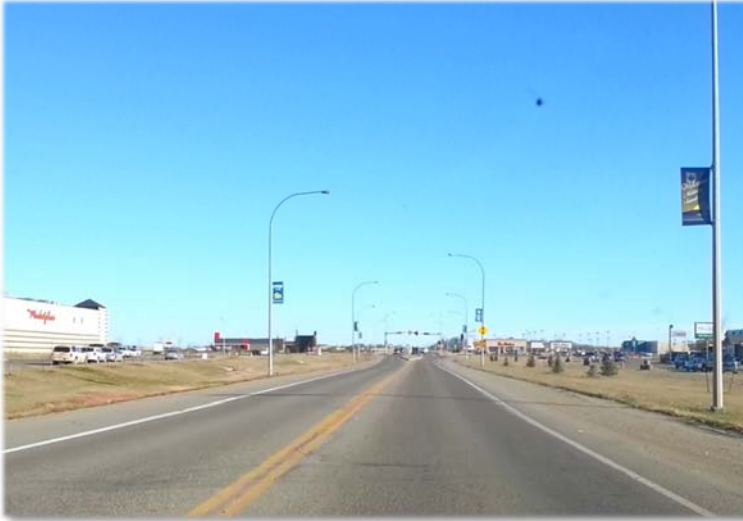
Photo 2-2: Highway 14 West of 23 Street, Looking East
